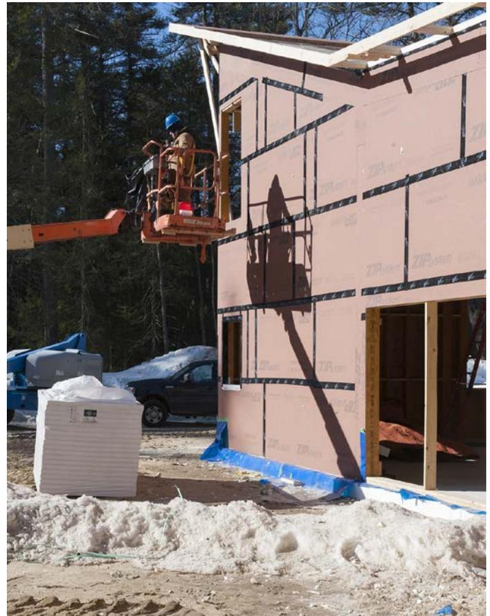
Airtightness was a high priority for the project, and the building turned out to be twice as airtight as Passivhaus standards require. Photo ©NCOB
