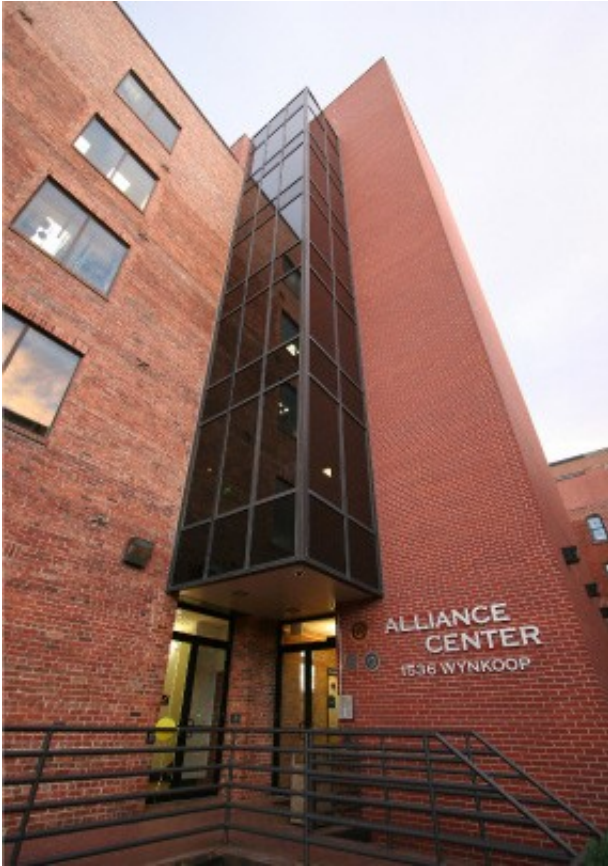
Exterior view of the Alliance Center
