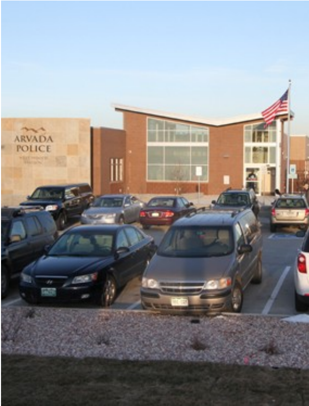
Exterior parking lot view
